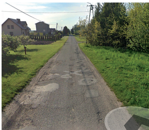
Fig. 13. Condition of the surface of road dr 1 before renovation
