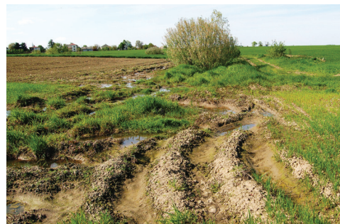
Fig. 4. Examples of badly located dirt roads – probably without prior analysis of water conditions
