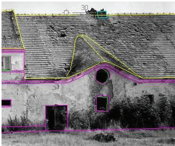
Fig. 1. Digitization of the object. Partially covered façade
