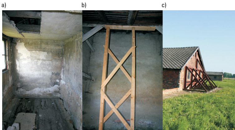
Fig. 1. The technical state of prisoner barracks in the former extermination camp Auschwitz II-Birkenau: a) the state of inner surfaces of load-bearing walls, b) inner supporting beam structure of the barrack, c) outer supporting beam structure of the barrack
