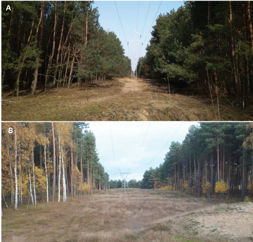
Fig. 1. Power line corridors within forest areas under single-rail lines of 110 kV in a triangular configuration (A), and 220 kV running flat (B)
